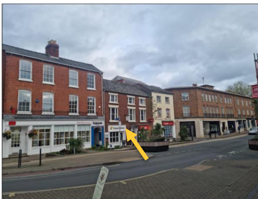
Plate 3: View looking NE from the corner of Bridge St and King St.
