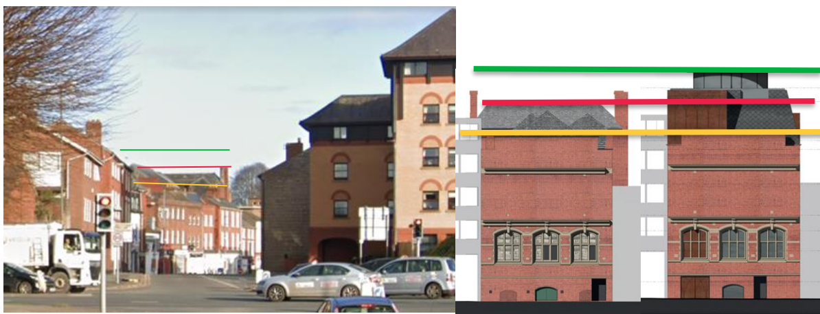
Photograph 22 from northern side of Barton Road illustrating gap
